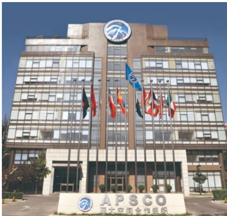
Photograph 5.1: APSCO Headquarters in Beijing (Source: www.apsco.int )
